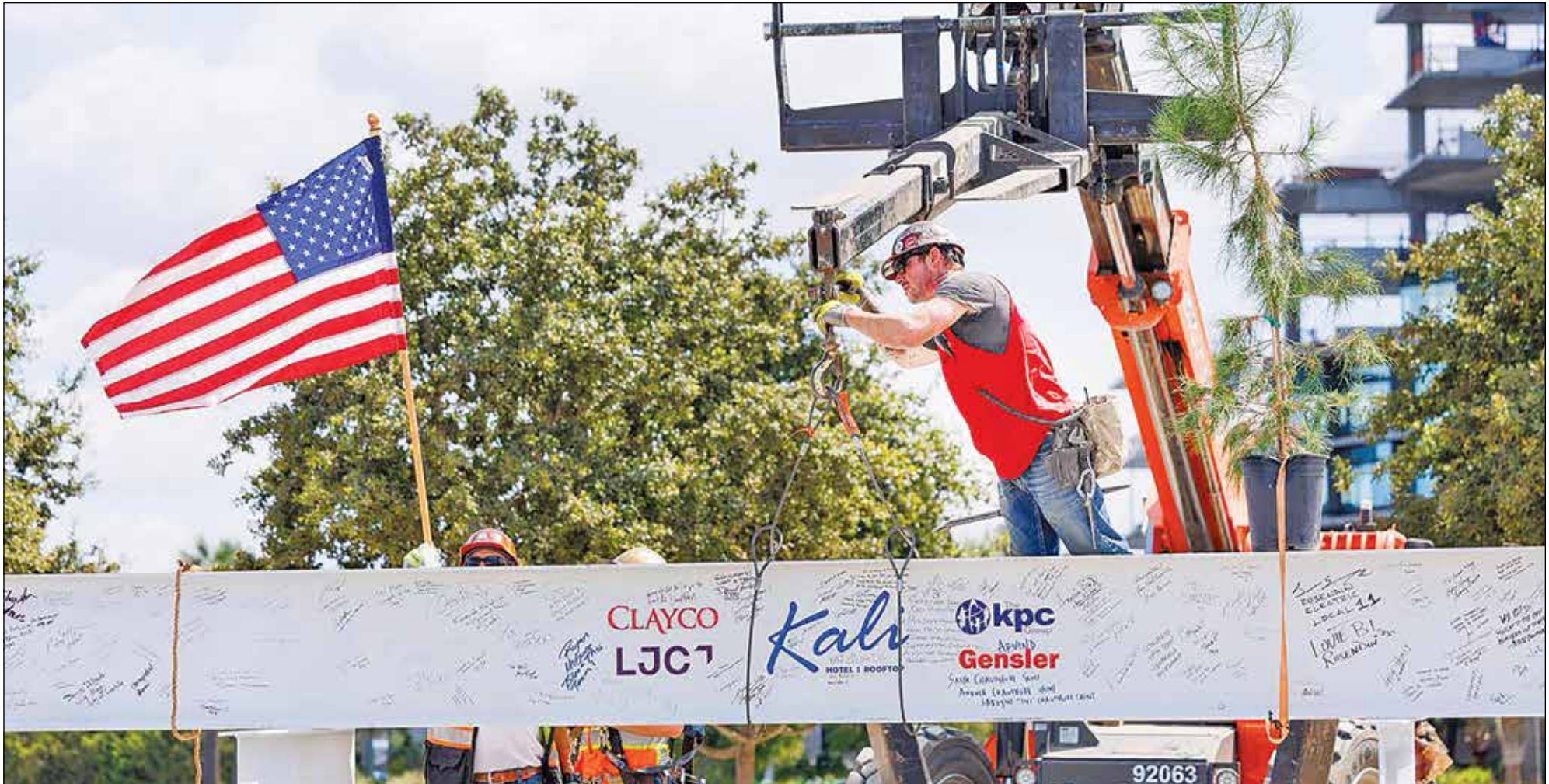
The ceremonial steel beam was raised, signaling completion of the building's structural frame. This new landmark will come to life ahead of premier sporting events in 2027 and beyond. Hollywood Park, where people can live, work, play and soon stay. Photo courtesy Hollywood Park Facebook page.
