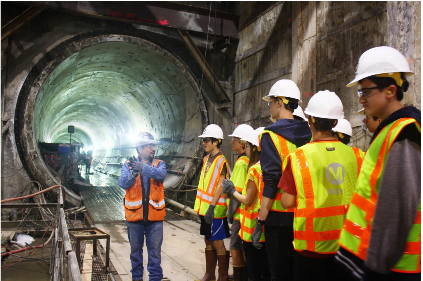
R.W. Carpenter, Tunnel safety Manager guiding El Segundo high school students through an overview of the tunnel during their tour of the Crenshaw/LAX Transit Project from Walsh Shea Construction Co.'s engineers
